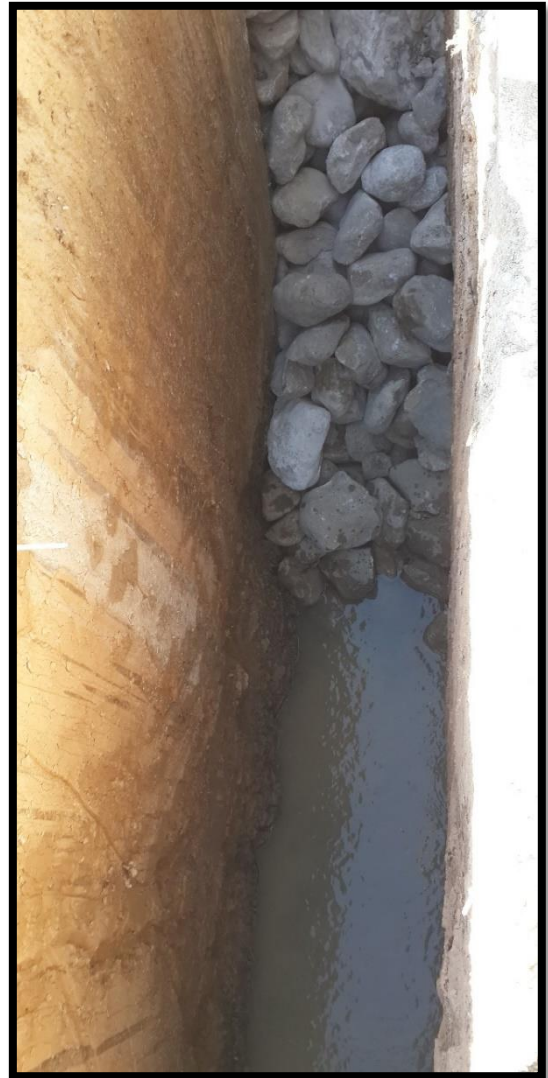
Picture 3 – Filling Excavating Channel by Boulder
