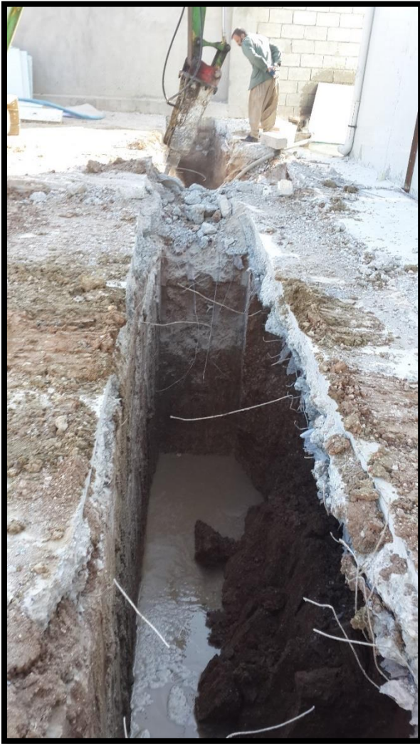
Picture 2 – Excavating Channel
