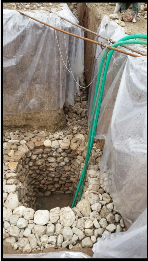
Picture 7 - Building a pool for collecting water and back filling by boulder.
